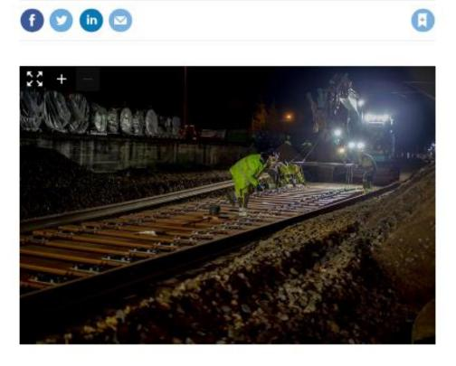
FINLAND: Transport infrastructure agency Väylä has started testing FFU synthetic sleepers from Sekisui on the 1 524 mm gauge national network, to assess their suitability for use in very low temperatures.
